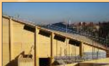
Figure 5: Kingsdale School, London by dRMM. CLT by KLH, with a 9 week build period.
