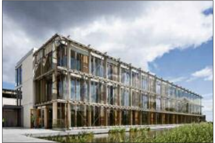
Figure 9: Ballyogan Environmental Management Centre 2012 by BucholzMcEvoy Architects. CLT by KLH
