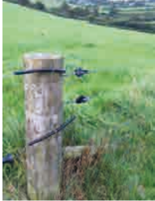
CCA treated fencing erected in 1995
