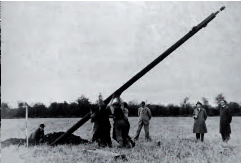
The first ESB transmission pole erected at Kilsallaghanlate, November 5th, 1946.
