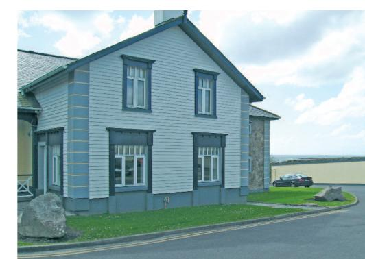
coating is required. Consideration should be given to the time of year when finishing is to be done and the oil content of the timber. For example, oily timber will delay the drying of oil based coatings. Also, when coated with water based finish, the air temperature will be a factor. Guidance should be sought from the coating manufacturer to identify the specific product to be used to give the desired finish and durability.
