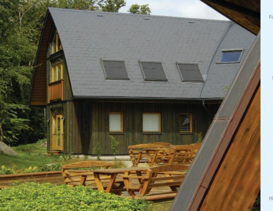
affected by moisture penetration and retention. Detailing of the substrate and the ventilation of cavities behind timber cladding should be designed to allow the back and face of the timber cladding to dry out at similar rates. All timber cladding should be installed with a ventilated cavity to allow the cladding to dry out evenly.
