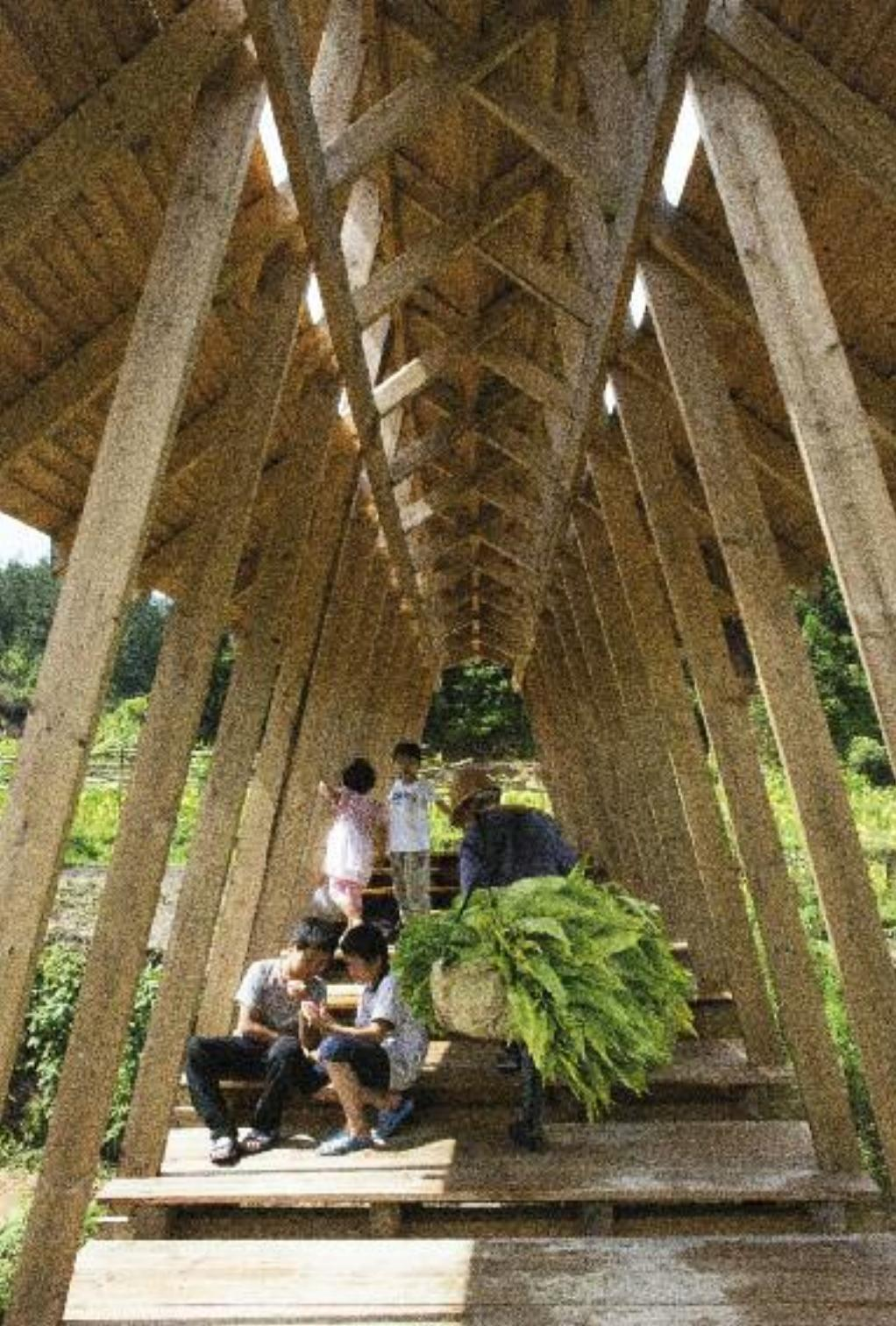
*Critical to this process was the integration of parametric digital design methodologies with more traditional construction techniques. BIM and CAD allowed for the planning and testing of complex assemblies before any handwork took place. CNC technologies was used to then create jigs and tools to enable rapid construction with unskilled labor and basic hand tools.*
