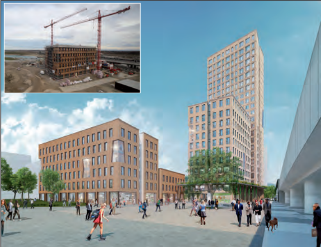
Artist's impression of 84-metre multi-storey building by Rüdiger Lainer and Partner (RLP), Vienna in engineered Norway spruce, which will save " 2,800 tonnes of CO 2 emissions over similar structures built in steel and concrete". Inset: the building under construction. Preliminary research carried out by NUI Galway shows that engineered Sitka spruce cross laminated timber (CLT) could offer similar benefits in multi-storey construction in Ireland. | RLP
