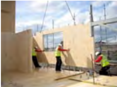
Figure 4: CLT wall element being lifted into place on the Murray Grove Building, London, UK
